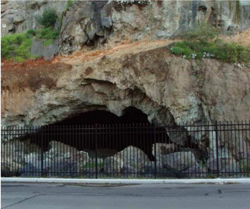
Moa Bone Point Cave after the major earthworks of 2016. Note the expansion bolts in the cliff above, trying to hold the rock together. This photo was taken before the footpath was re-instated with the only real way to view the cave being from across the road. Photo: M. Traves, May 2017
