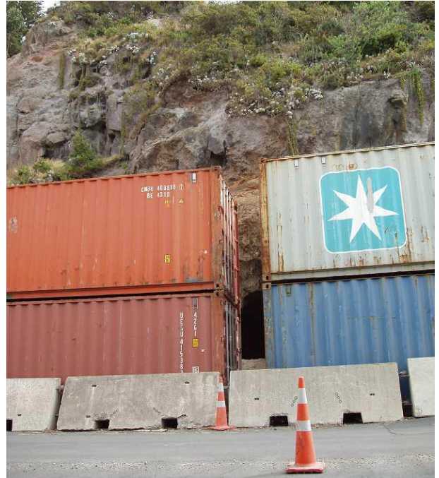
By December 2011 there was a double stack of containers lining the roadside all along the cliff areas on the way to Sumner. Moa Cave is just visible between the containers – it remained blocked off like this for about four years!
